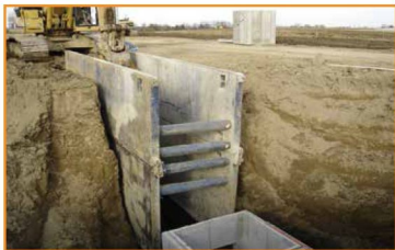
Stacked Trench Shields
