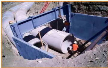
A 6M Series Trench Shield with Height Adapters
